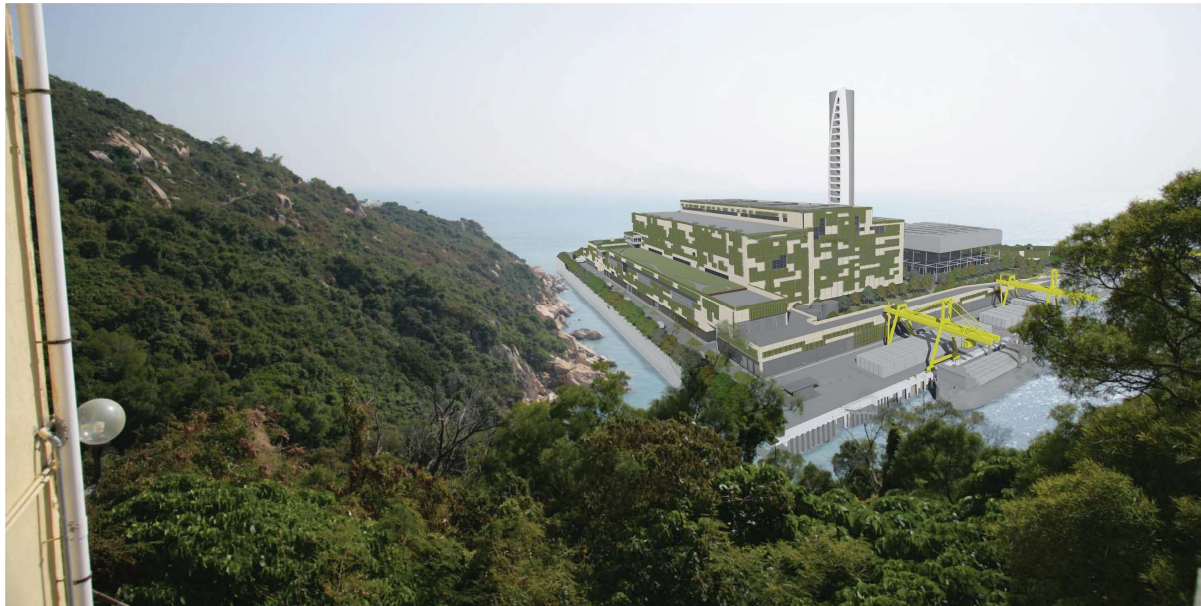
VSR 3 Administration and Residential Building Cluster
