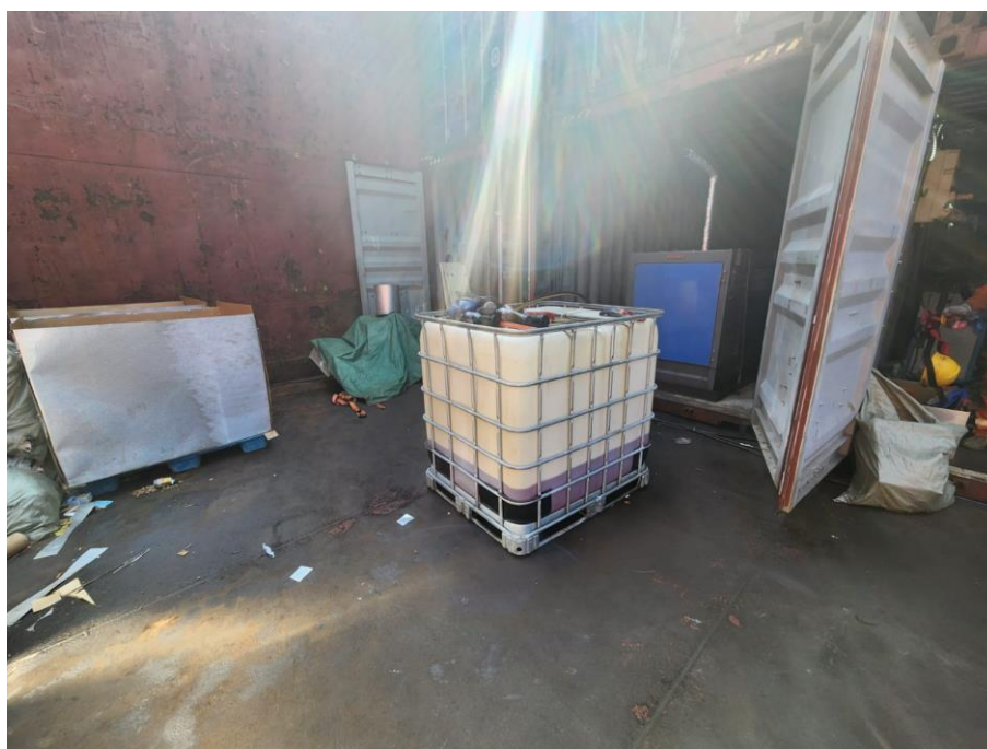
Figure 5: Site Photo of Container for Diesel Fuel Storage Taken during the Inspection on 10 January 2025 by SO and the Contractor
