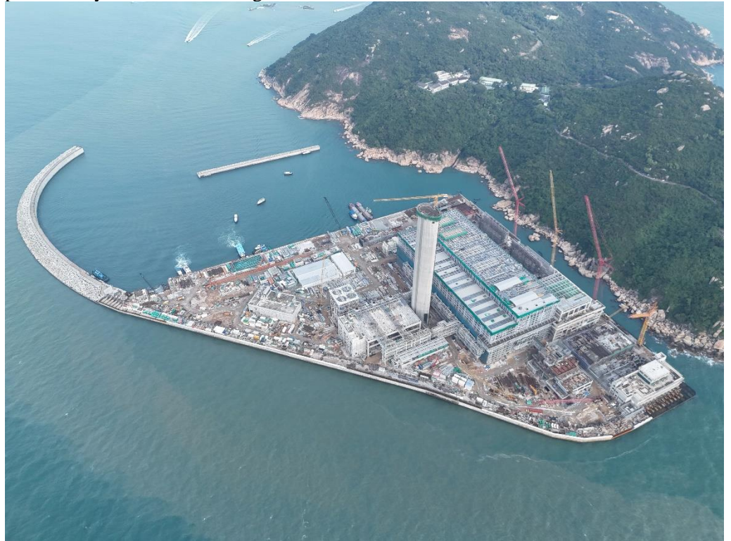
Aerial Photo Record of the Project Site
