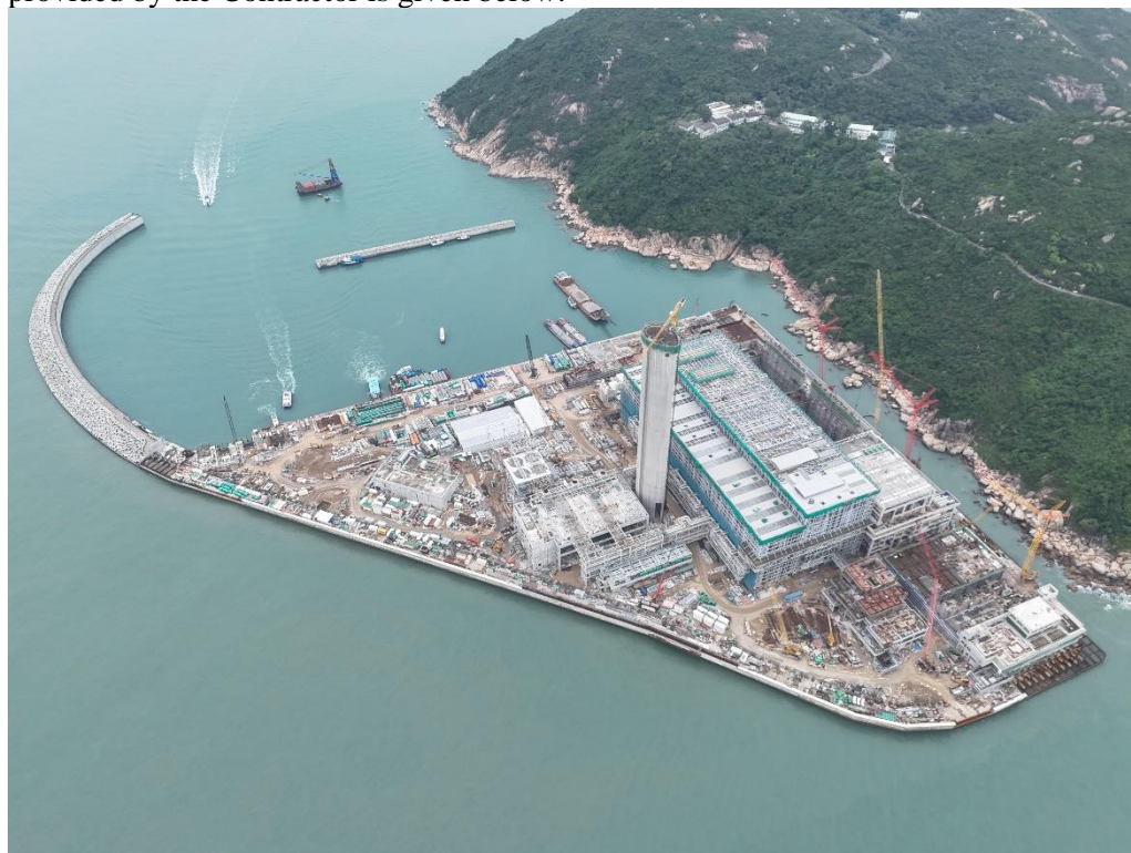
Aerial Photo Record of the Project Site
