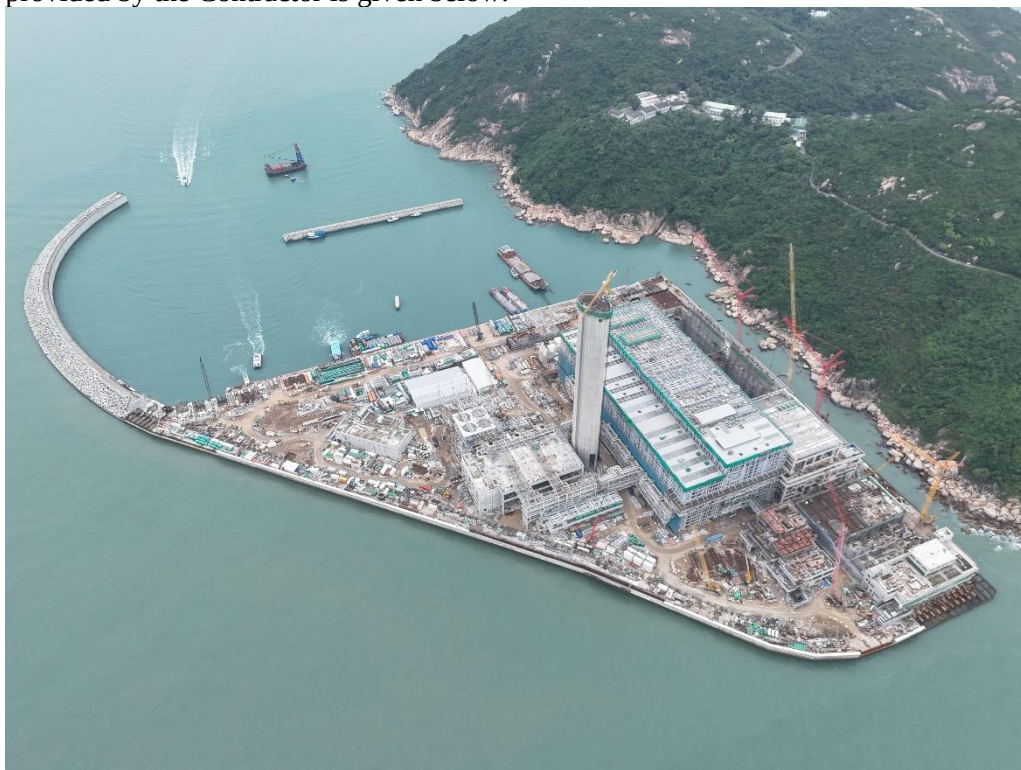
Aerial Photo Record of the Project Site
