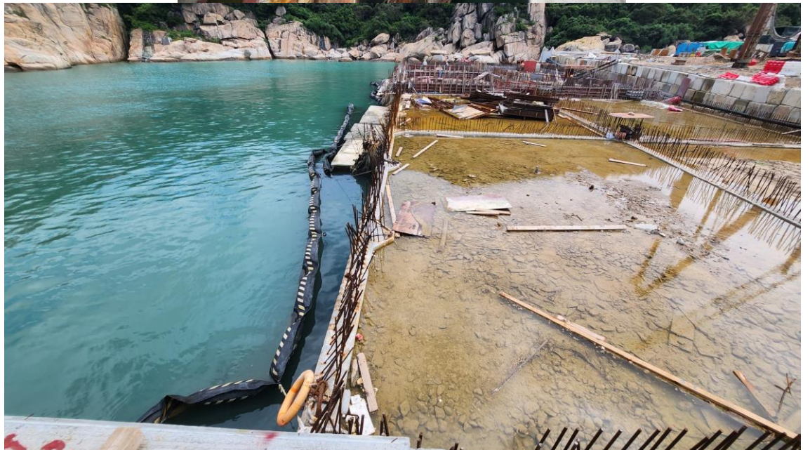
Figure 4 Shore Condition along Seawall B during Site Inspection on 19 September 2023
