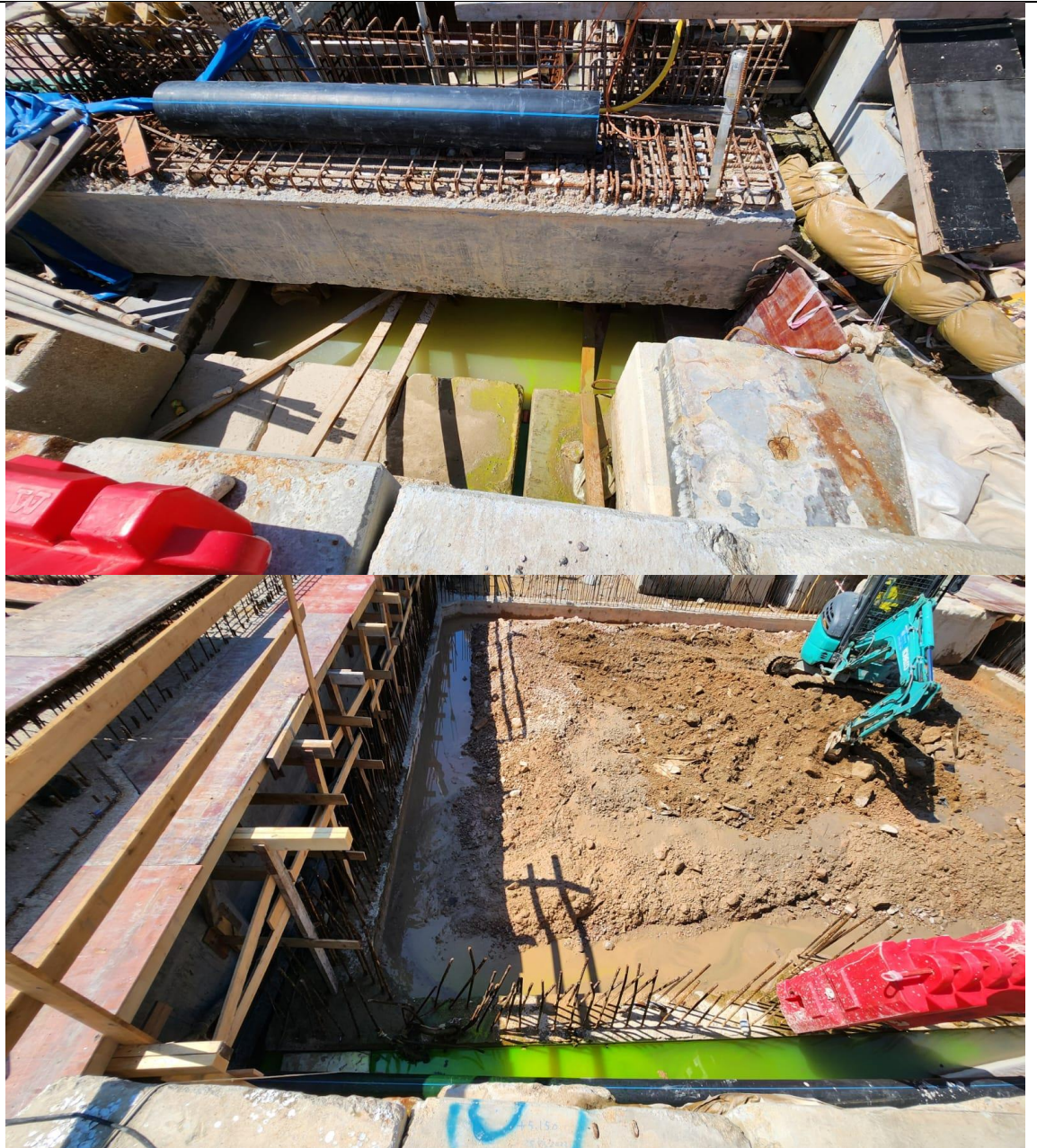
Figure 6 Leakage Test at Caisson 5 and Caisson A2
