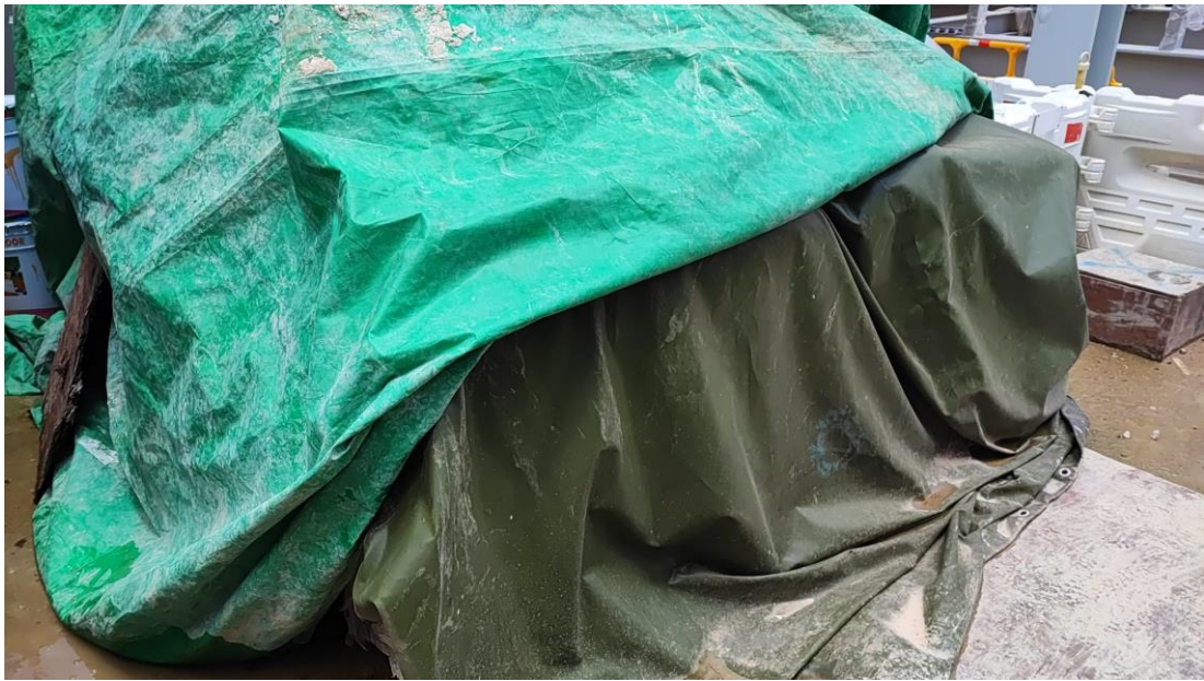
Figure 8: Photo Record of Covering Dusty Material with Impervious Sheet Entirely
