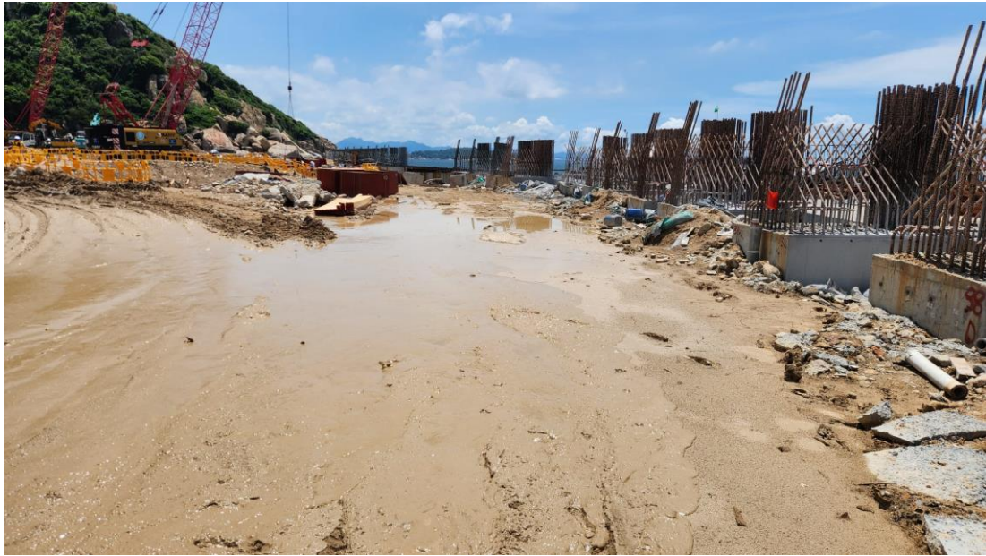
Figure 4: Site Photo of Main Haul Road Taken during Site Inspection on 12 June 2023
